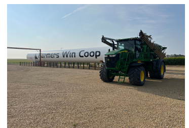
Jackson Junction NH3 Site
